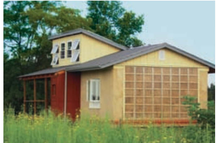
The Eco Center, constructed from straw bales, is a hands-on laboratory where students can research and develop sustainable practices.
