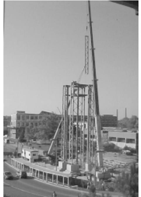
In early October the steel framing is well under way. The first level of steel has been placed on the concrete bases. It is approximately 80 feet high. The crane is lifting the first of four upper-level corner pieces. In the foreground, protective covering has been installed over the sidewalk to shield pedestrians from small falling objects.
