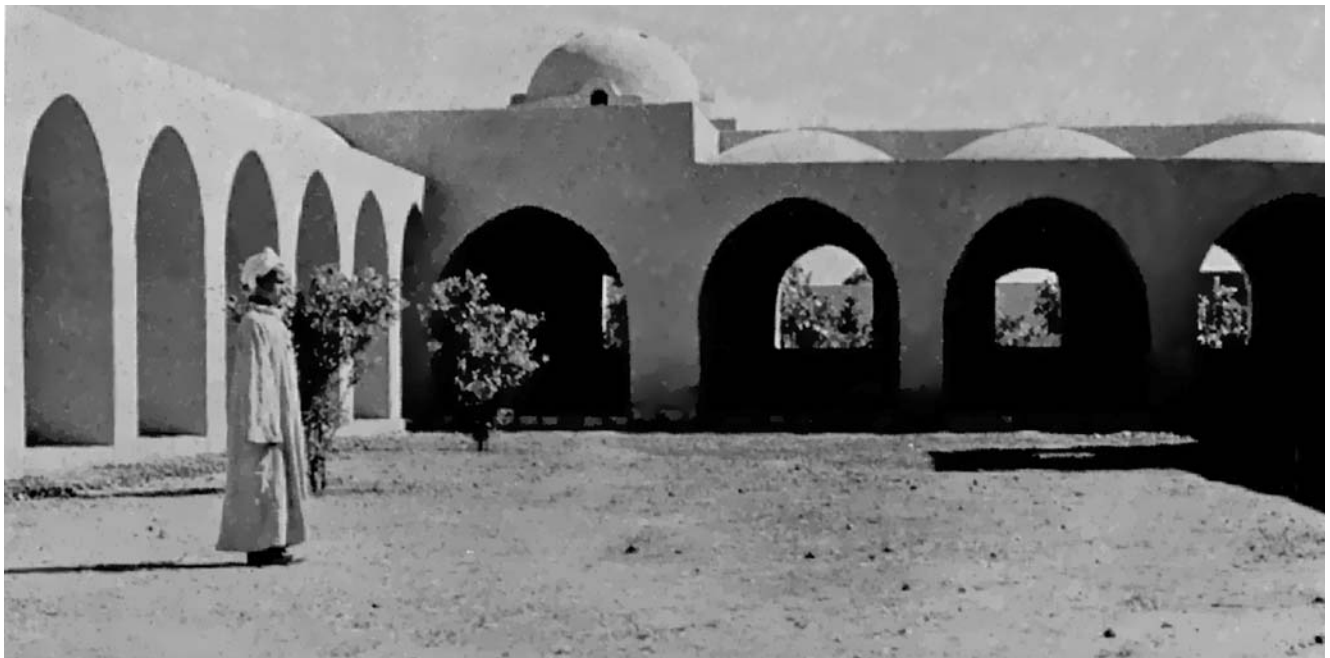
Fig. 40.1 Traditional masonry structures in Egypt
