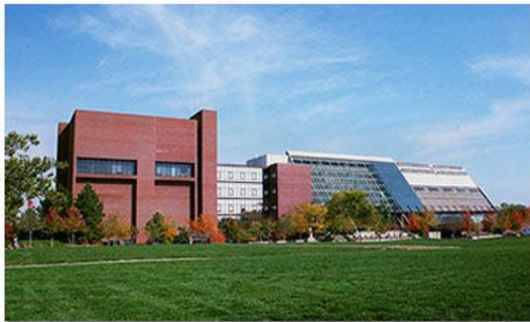
In our building (AB)
