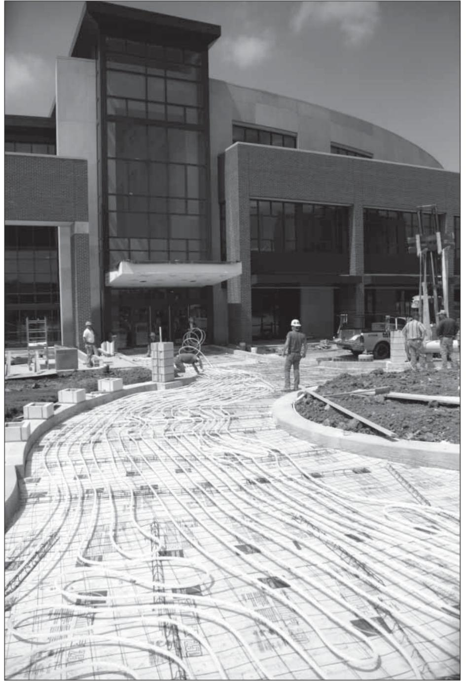
Heated piping runs beneath the entryway to the new Communication and Media Building set to open for the Fall 2007 semester. Photo by Doug Blemker
